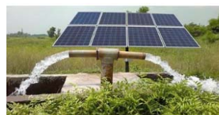
Groundwater pumping system (using Solar energy)
