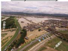
(5) Flood damage caused by Odagawa River (Kurashiki City, Okayama Pref.)
