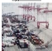
(6) Flood damage at Rokko Island, Port of Kobe (Kobe City, Hyogo Pref.)
