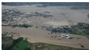
(1) Flood damage due to embankment collapse of Kinugawa River (Joso City, Ibaraki Pref.)
