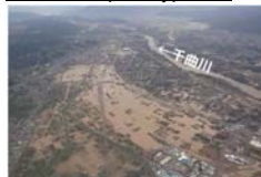
(9) Flood damage caused by Chikuma River (Nagano City, Nagano Pref.)
