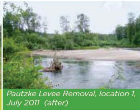
After removing levee
