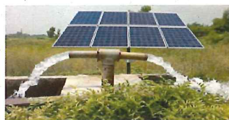
Groundwater pumping system (using Solar energy)
